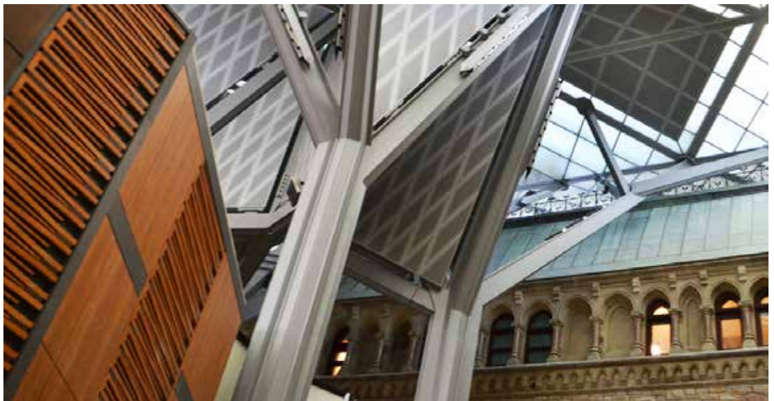
West Block, Parliament of Canada, Complete Restoration, Rehabilitation and Addition, Ottawa, ON
