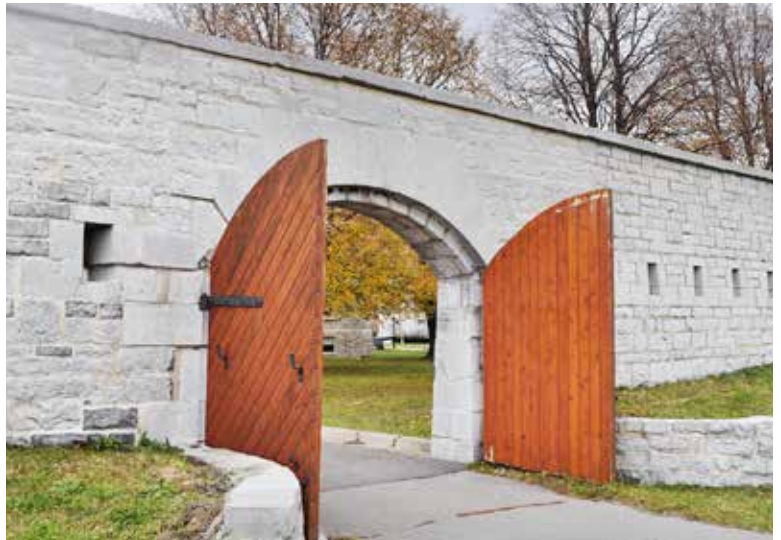
Fort Frederick, Restoration of Fortifications Wall and Martello Tower, Kingston, ON
