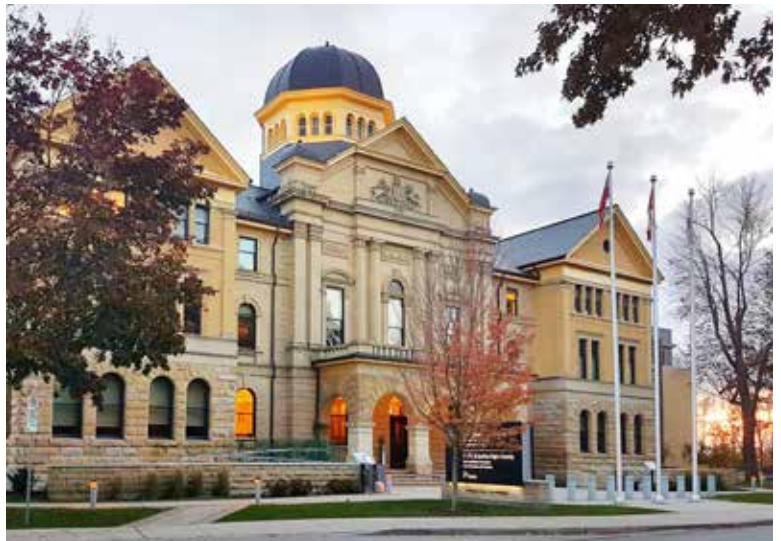
Elgin County Courthouse, Complete Restoration and Rehabilitation, St. Thomas, ON
