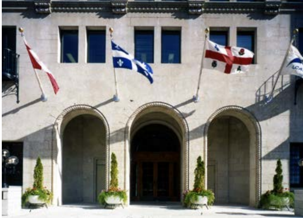
Rehabilitated front facade of the Berkeley Hotel once the canopy / bar was removed. The three arches were opened up to create ground floor loggia and to disguise the fire exits onto Sherbrooke street.
